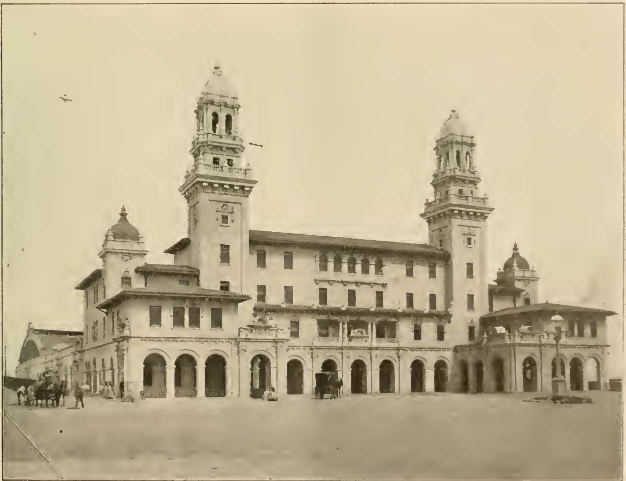
ATLANTA'S NEW TERMINAL STATION.
